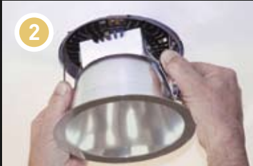
Put Torsion Springs Into Brackets
